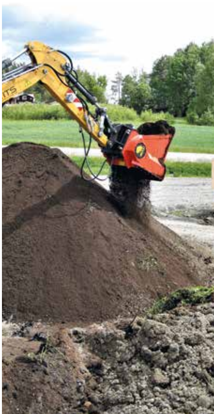
ABOVE: Kits Contractor in Sweden uses ALLU attachments for the recycling of construction waste
